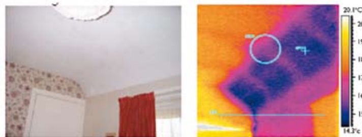
Figure 39: The missing loft insulation near the eaves.
